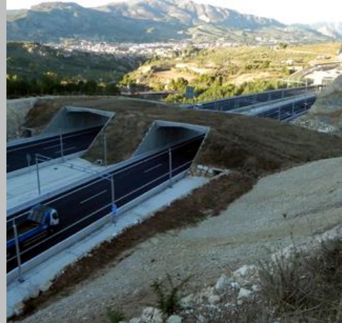
Photo 2 - Overpass details (© J. Juste)
