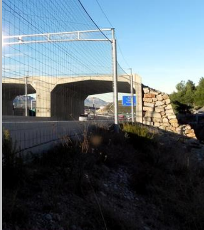
Photo 1 - Detail of the net that covers the A7 in the vicinity of the bat shelter (© Miguel Angel Monsalve)
